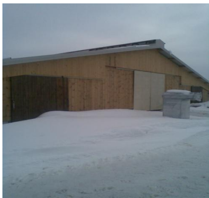
The cattle barn renewed in 2010, Photo UL, Slovenia
