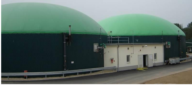
The farm anaerobic digester
